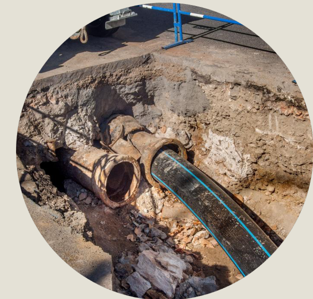
Sewer Connection Grants
